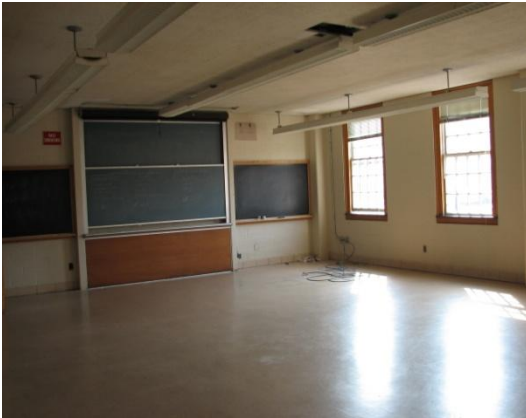
Rosenau 228 Before Renovation
